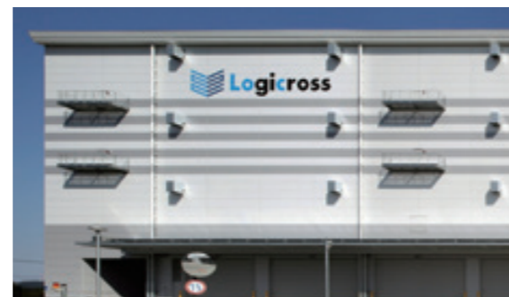
Insulated sandwich panels for exterior walls
