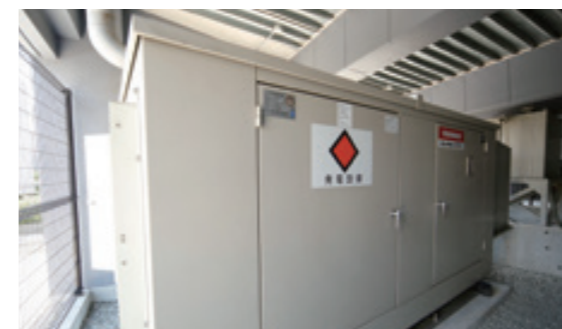
Installation of emergency power generators
