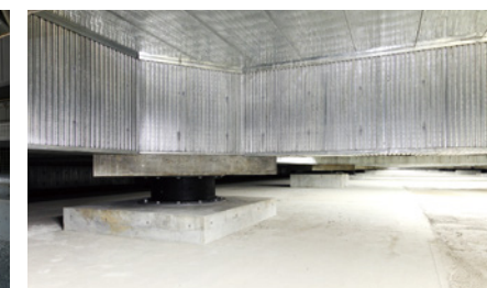
Seismic isolators
