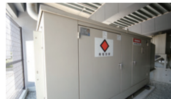
Installation of private power generators
